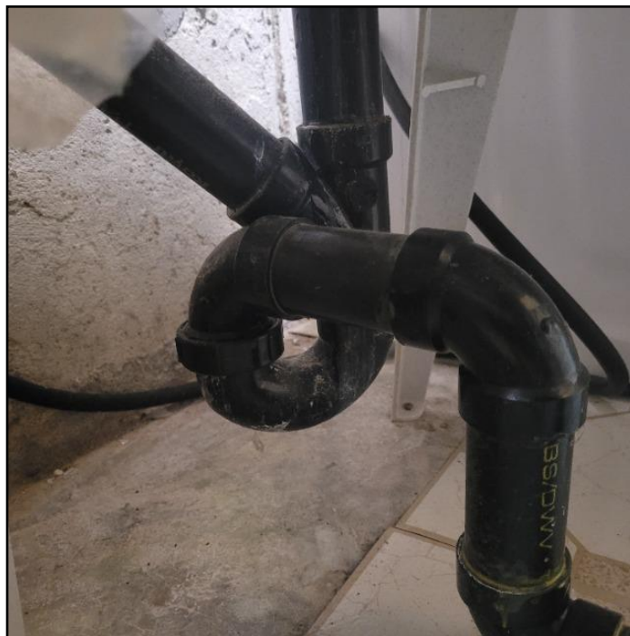
11. Nonstandard trap installation
