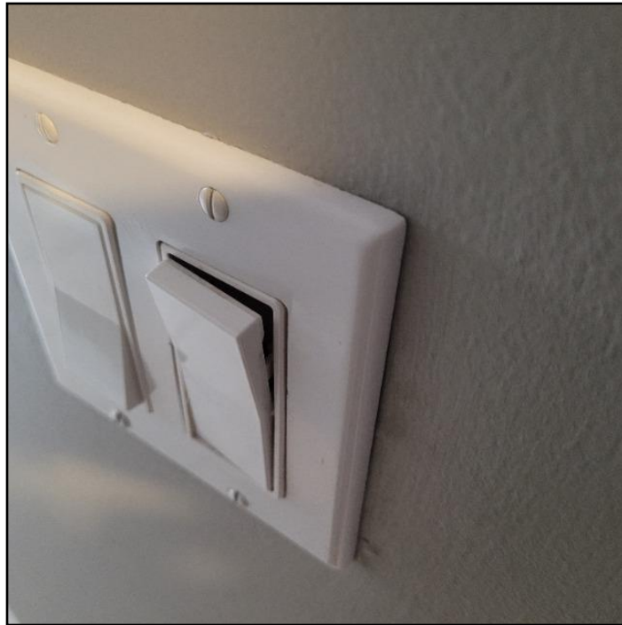
7. Damaged switch
