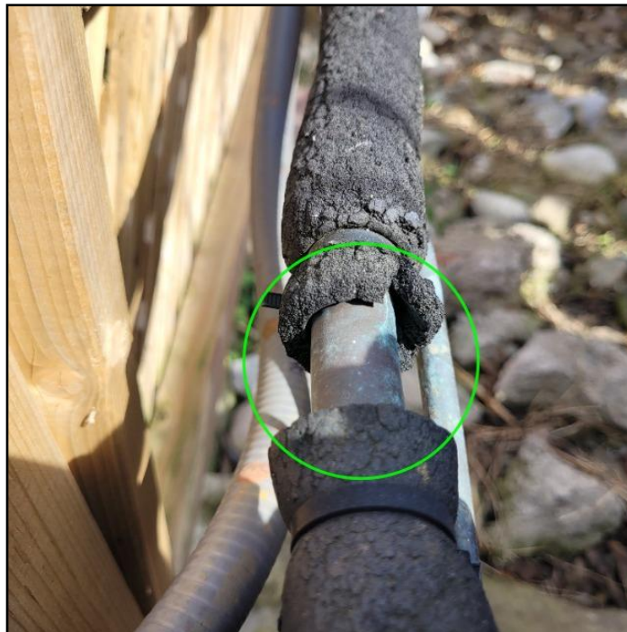
10. Insulation - missing
